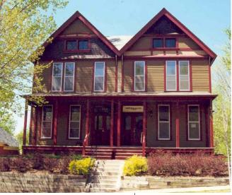
735-737 E. 5th Street, before photo at left, after photo above showing reconstructed front porch, restored siding and an appropriate paint scheme.
